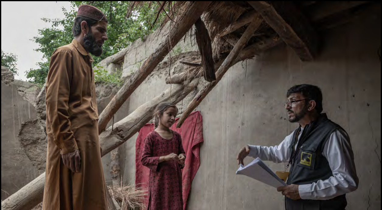
Baryalai, an IRC humanitarian access officer, speaks with Azim Khan, 35, and his daughter Bibi Zainab, 9, about the damages caused to their home due to heavy rains and flooding that impacted 32 out of the 34 provinces in Afghanistan.
